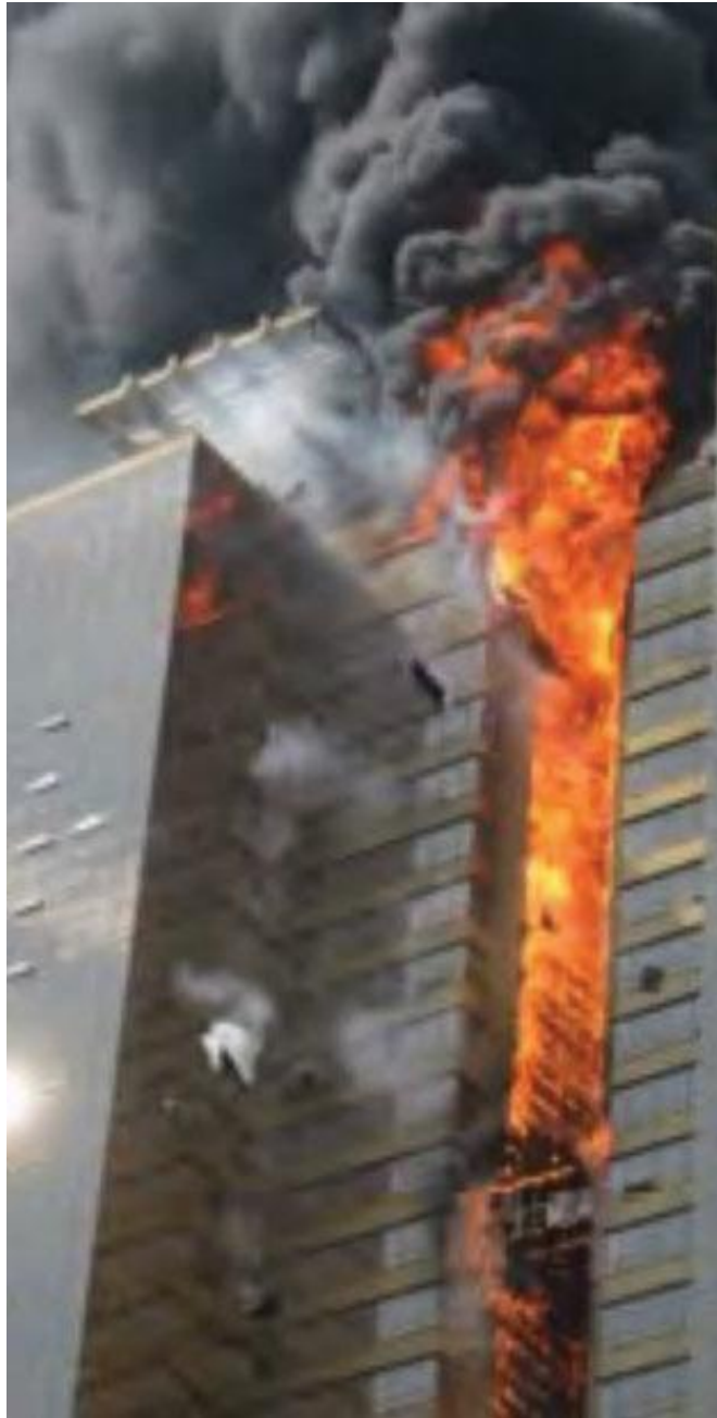
In Wooshin Golden Suites Busan, South Korea (1) , a vertical, U-shaped channel enhanced fire spread through reradiation and chimney effect.
